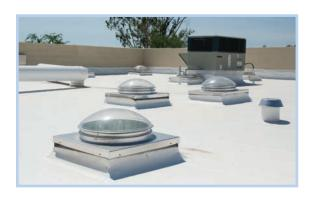
Dark warehouses and commercial office buildings are no match for Natural Light's tubular skylights. Installed on virtually any type of roof surface in under two hours, our 21" commercial units are capable of delivering up to 1400 watts of light without the heat gain or heat loss of a standard framed-in skylight.
